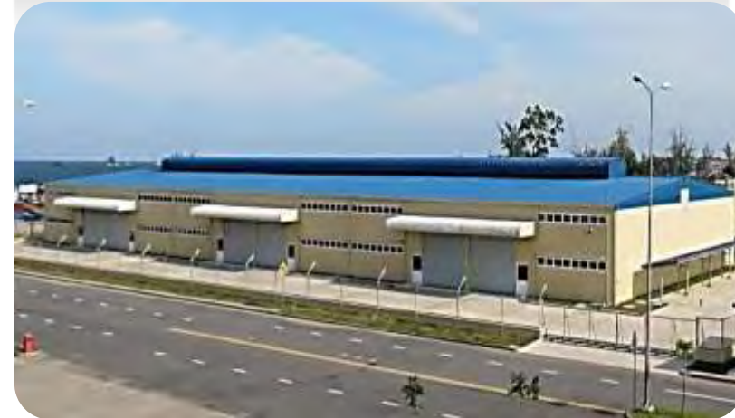
SPSEZ Rental Factory (2,700m 2 ) 1,650m 2 Occupied by Oji & 1,050m 2 Occupied by IS-TEC
