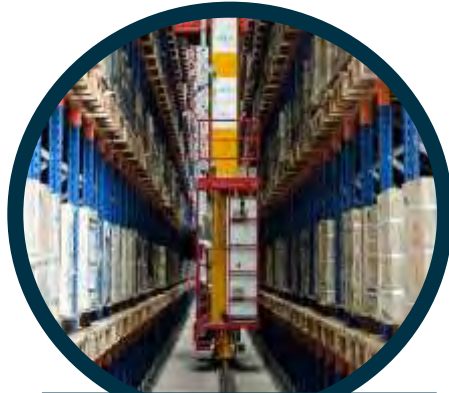
Automated Storage and Retrieval System
