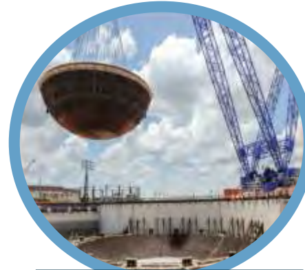
Super Heavy Cranes
