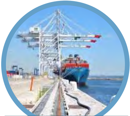
STS Crane Runways and Trolley
