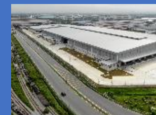
Northport's three new warehouses equipped with solar panels, with 350k sq ft area began operations in Oct 2021
