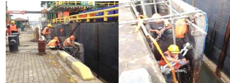
Installation of new Chain System
