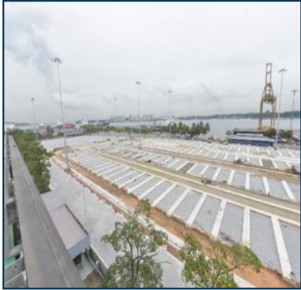
NEW YARD AREA
