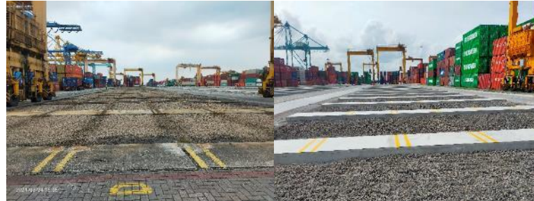
Rehabilitation of Container Stacking Beam
