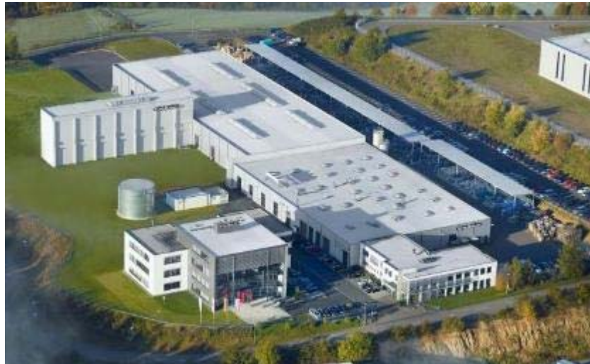
TSUBAKI KABELSCHLEPP Headquarters Wenden, Germany
