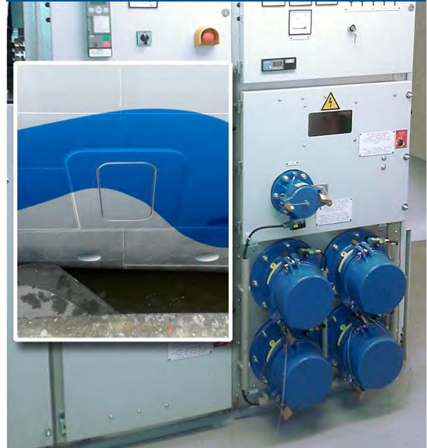
Ship's hatch / Control Cabinet
