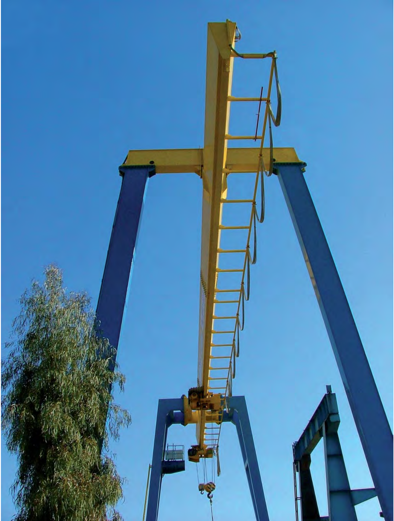
Poolad Crane Co. – Gantry Crane 50-Ton – Length of Girder 36 meters
