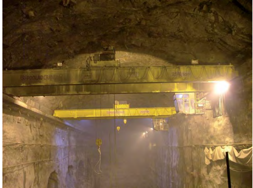
Gotvand Dam Kian Payab EOT Cranes 2x20(40)Ton 2 Sets
