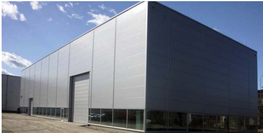
Electrical Hall, Eberswalde
