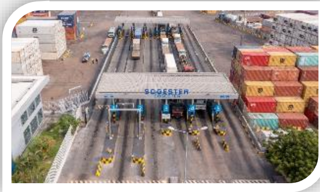
Gate Automation Camco OCR system (pilot Go-live)
