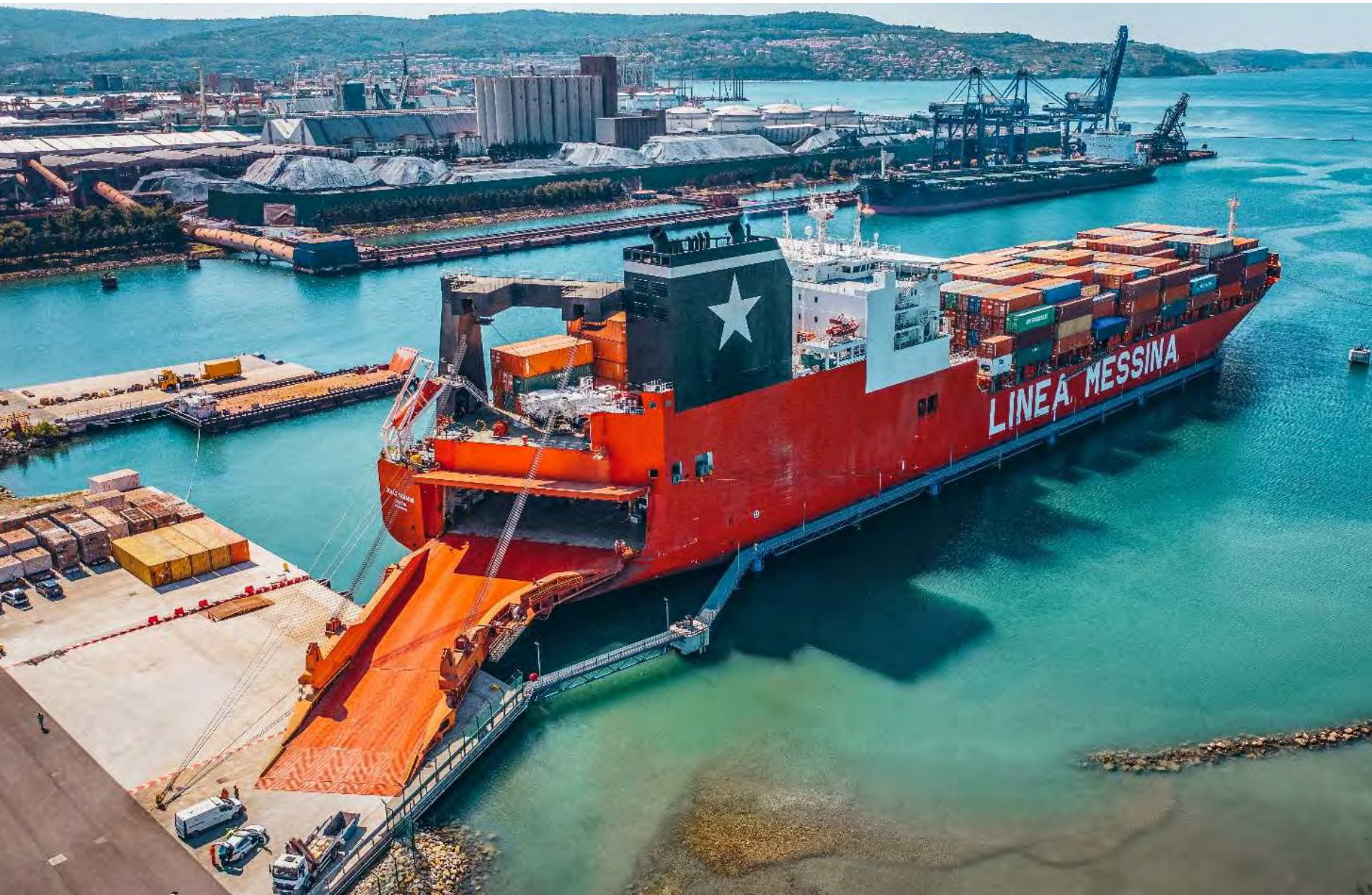
New dedicated RO-RO berth
