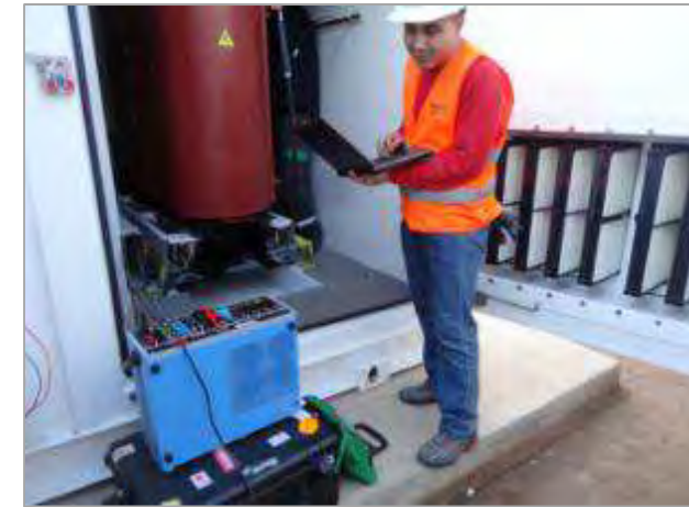
During the commissioning, end of January 2014
