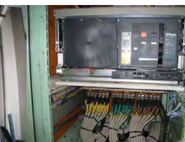
Shore in-come CB Synchro module Switch board adaptation
