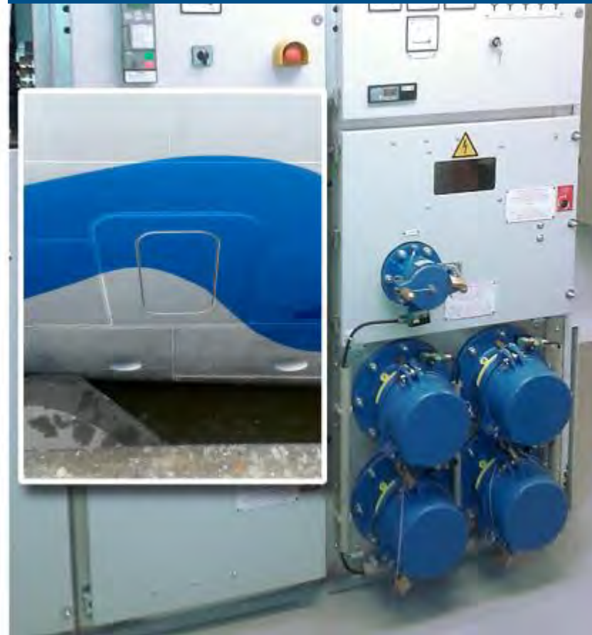
Ship's hatch / Control Cabinet
