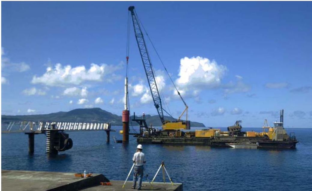
Construction of dolphins - Fort de France Muriers Cove breakwater - Guadeloupe
