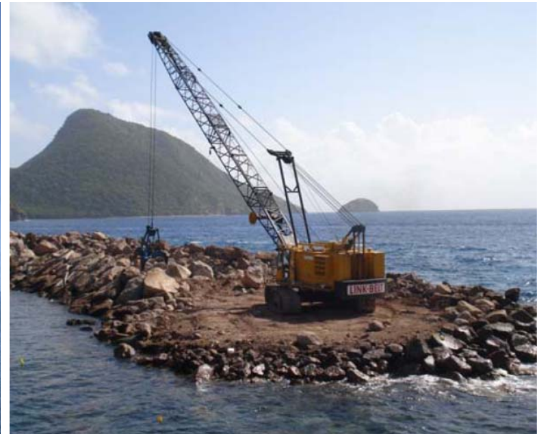
Construction of dolphins - Fort de France Muriers Cove breakwater - Guadeloupe
