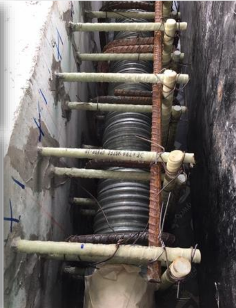
Concrete with GFRP dowels & post-tensioned steel bar
