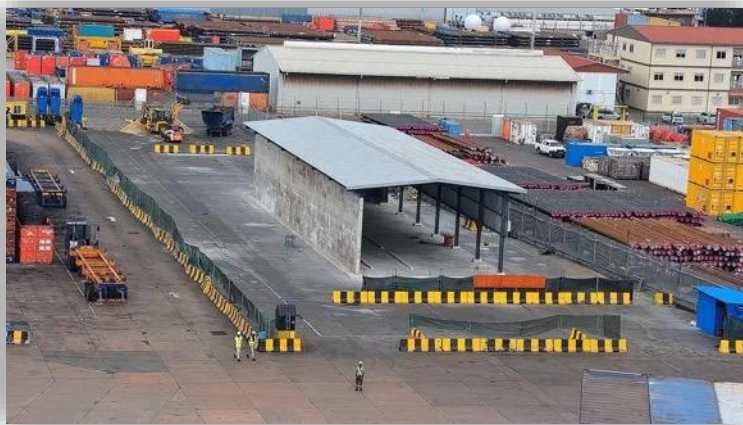
X-Ray Scanner – under construction, Nov.2024
