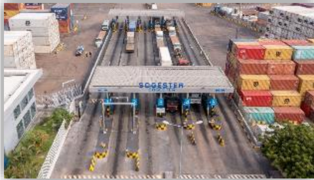
Gate Automation Camco OCR system + Pin stations OCR
