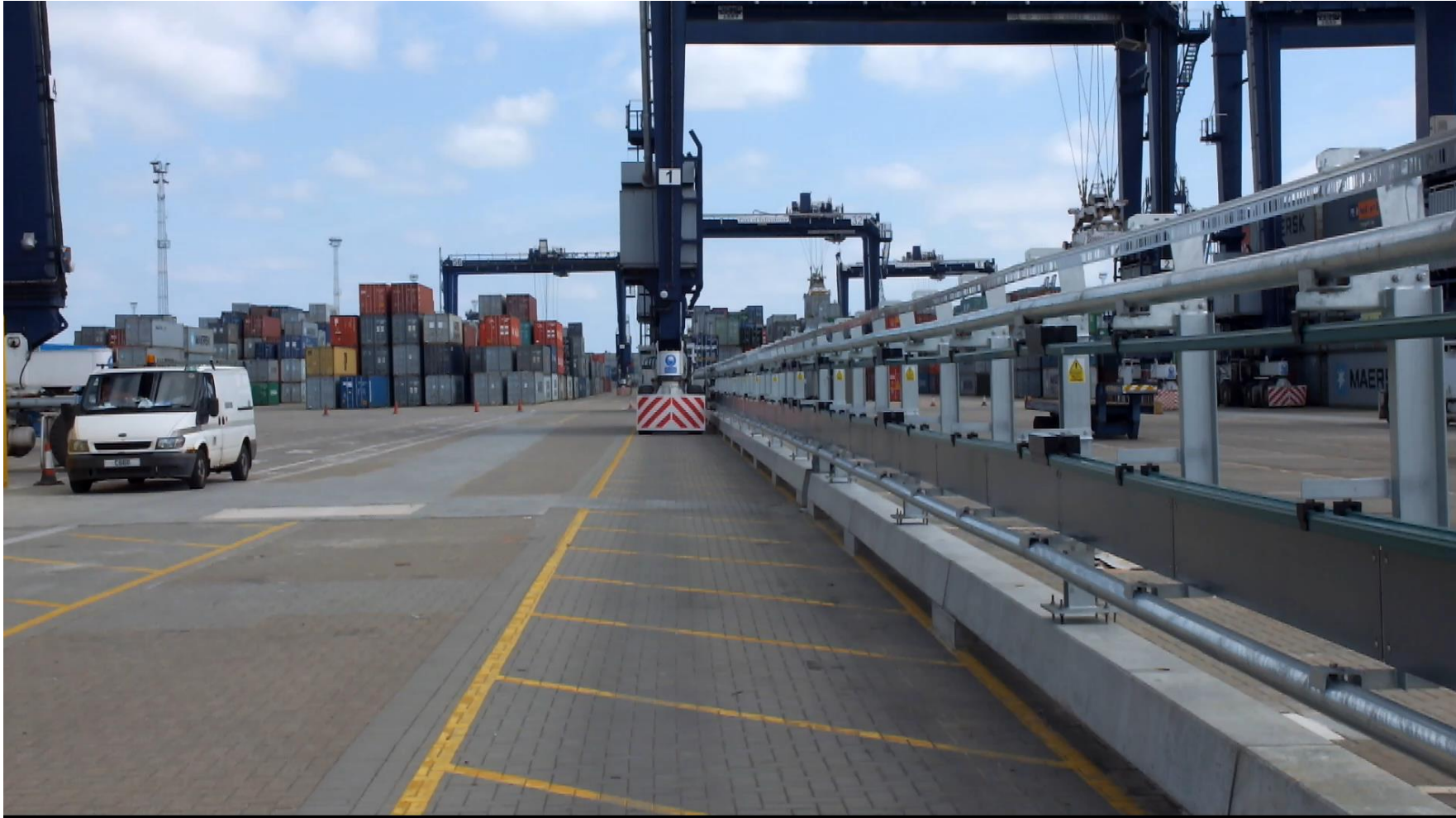
Retrofitted ZPMC RTG crane Siemens PLC: Autosteering with up to 160m/min
