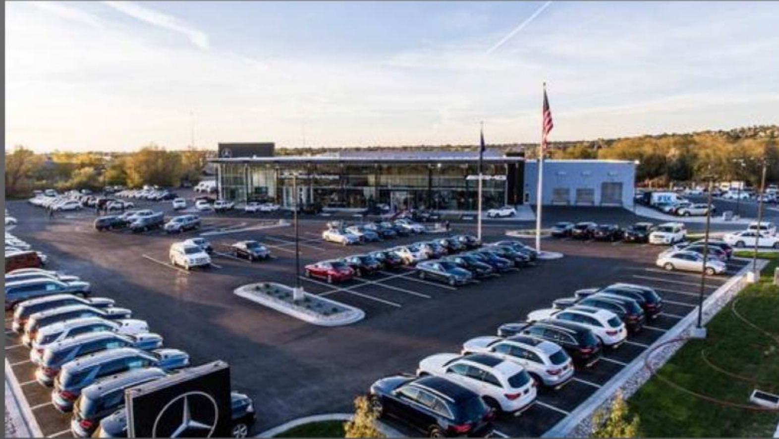
Scaling physical barriers into semi-fenced business facilities
