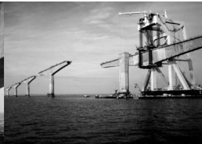
Confederation Bridge Canada
