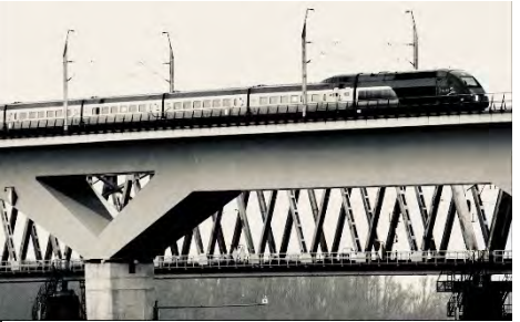
Hollands Diep High Speed Rail Bridge The Netherlands
