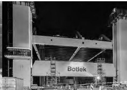
A15 Botlek Bridge The Netherlands
