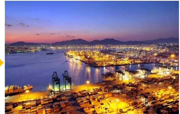
SAPANGAR BAY CONTAINER PORT
