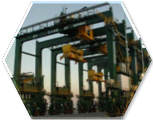
DC power supply bridge
