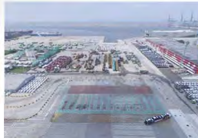
LOADING/ UNLOADING AREA CAR CARRIER
