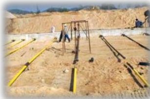
Preparation of bars
