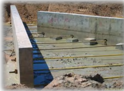
Anchoring plates to mailand
