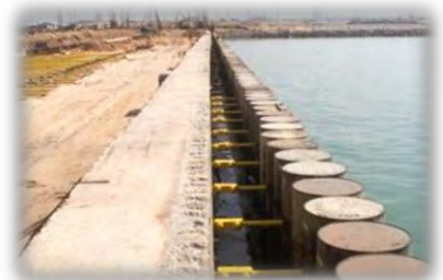
Load full completed
