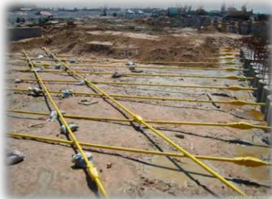
Preparation of bars
