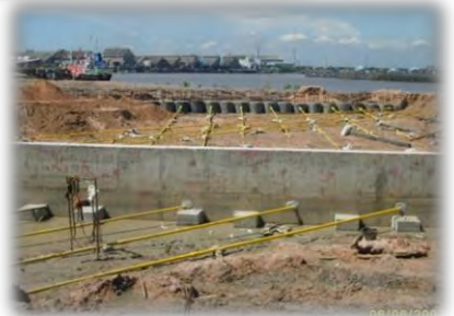
Bars connection through wall
