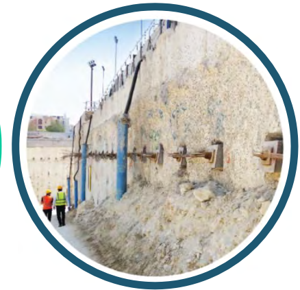
Ground Engineering Solutions
