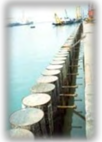
Anchoring piles connected
