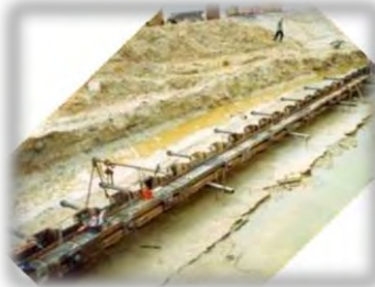
Retaining wall completed
