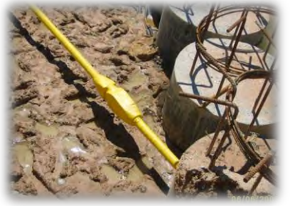
Anchoring piles connected
