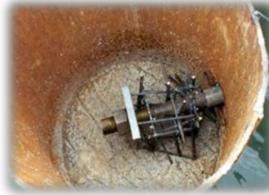
Preparation of anchoring pile
