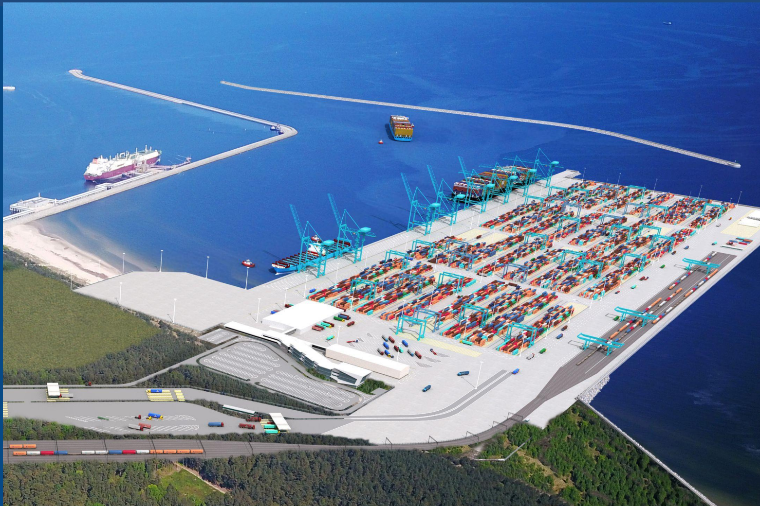
New deepwater container terminal in Świnoujście
