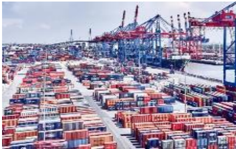
Container Terminal Burchardkai
