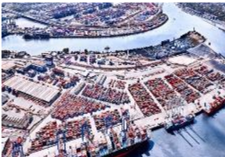
Container Terminal Tollerort
