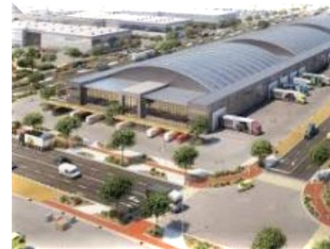
Integrated storage zone with a land area of 74.9 ha for development of integrated industry
