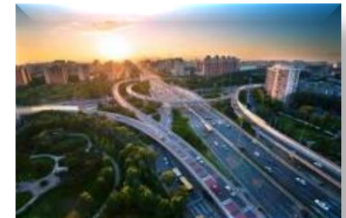
Construction of urban highways
