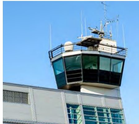
ELECTRONIC NAVIGATION, AIS & MONITORING
