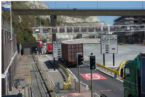
Traffic control and monitoring systems
