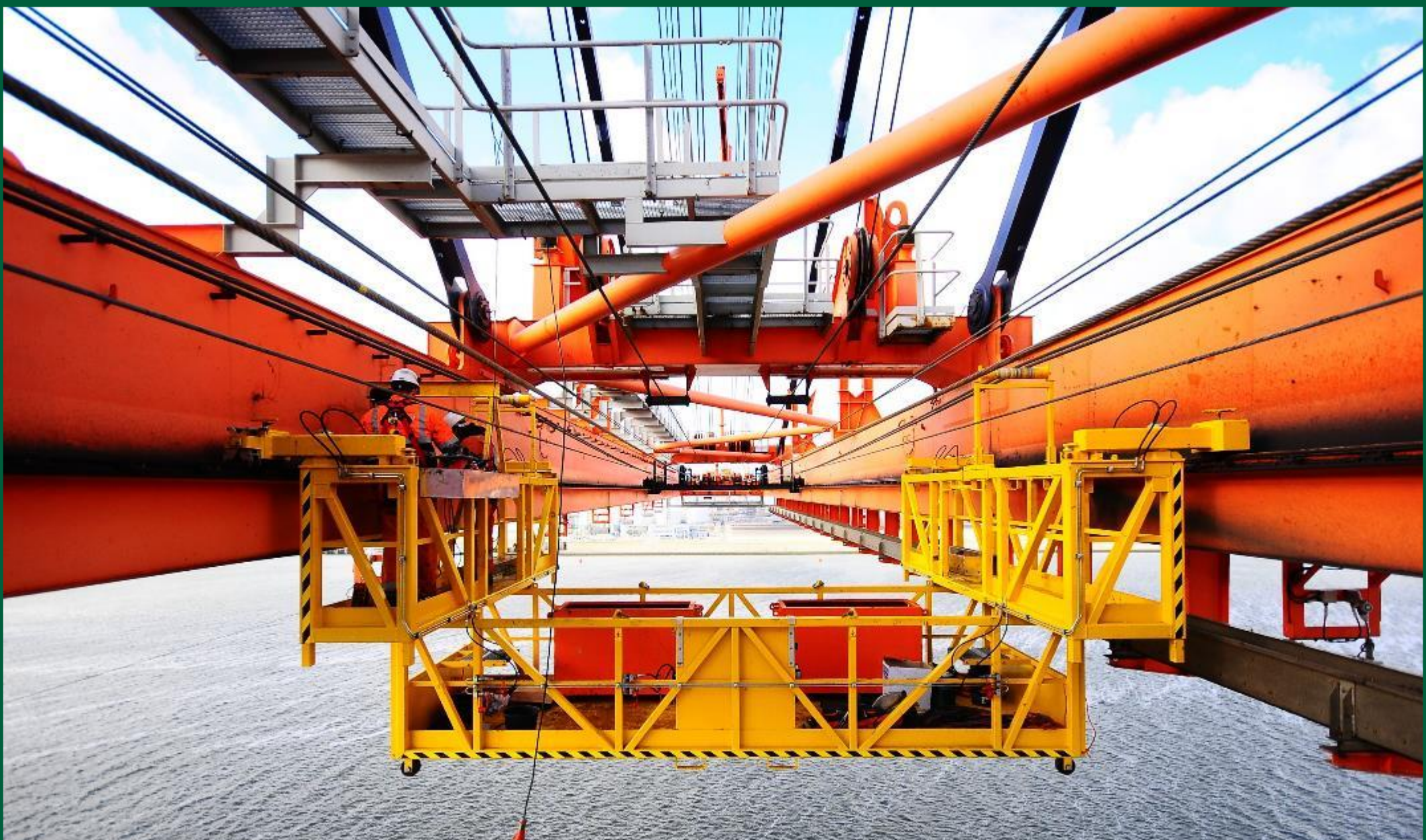
Bemo Rail Maintenance platform supply and installation – trolley rails
