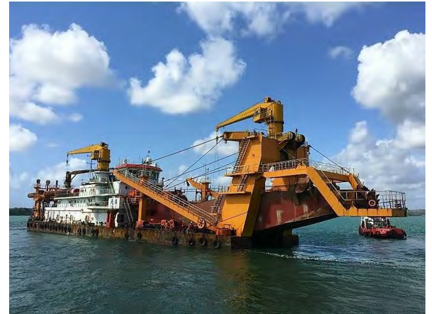
Ongoing Dredging Works
