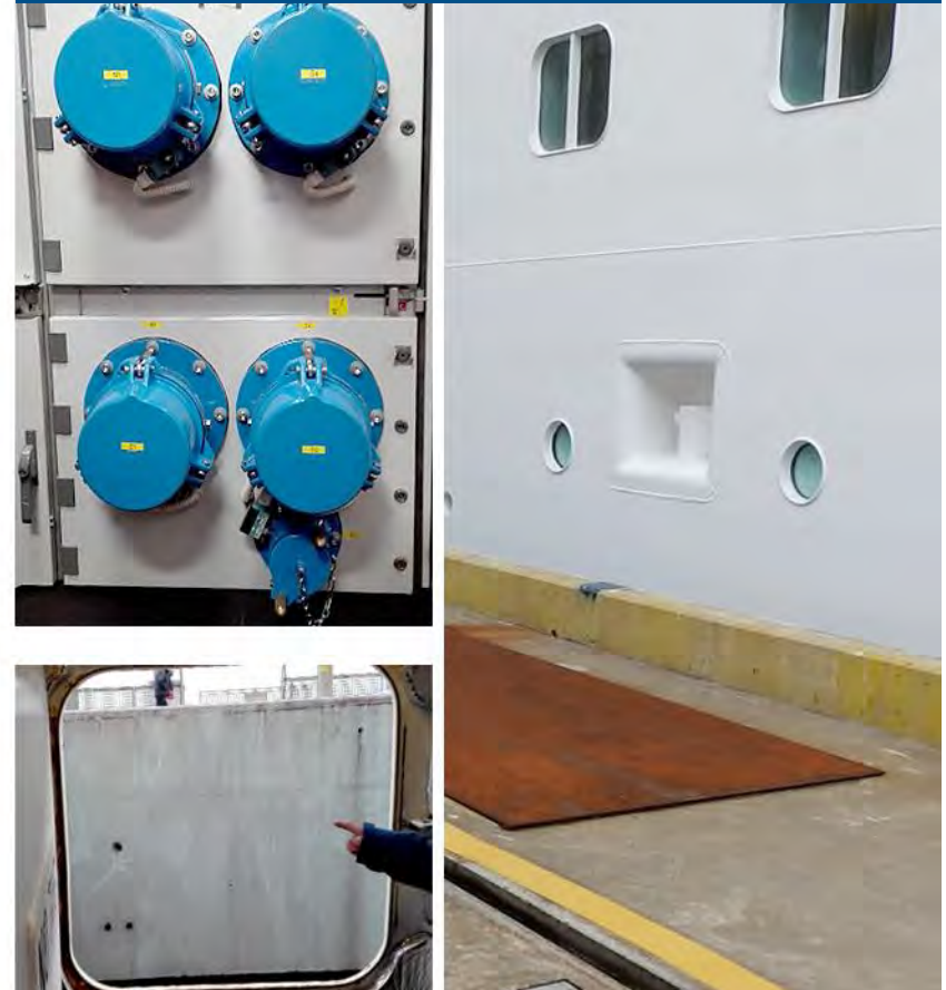
Ship's hatch / Control Cabinet
