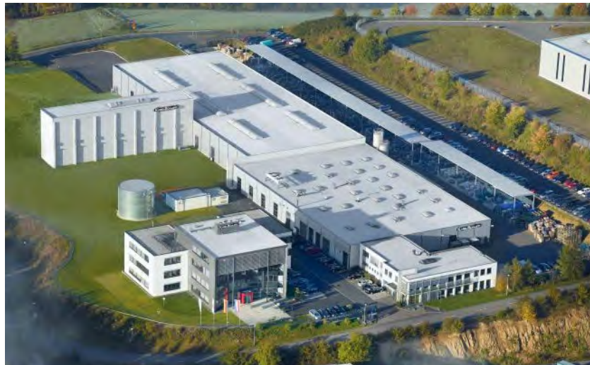
TSUBAKI KABELSCHLEPP Headquarters Wenden, Germany
