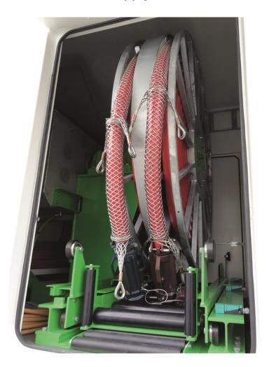
The feed of the onshore power supply for container vessels is realised for example by the installation of a 40 ft. HC-container in the bottom storage row.
