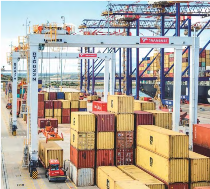
Stacking: Rubber tyre gantry cranes
