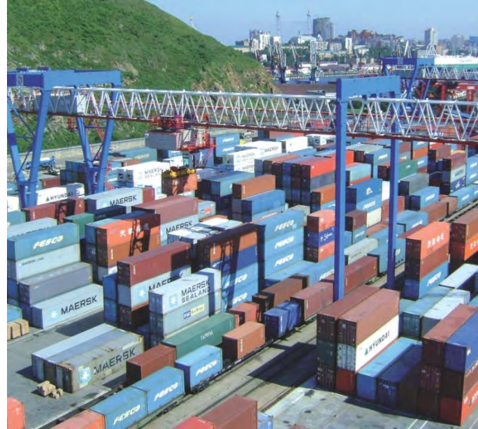
Stacking: Rail mounted gantry cranes
