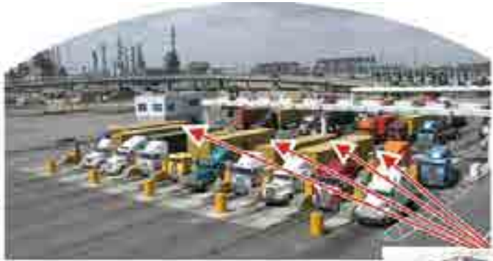
Automatic Gate-in inside the port area thanks to RFID antennas
