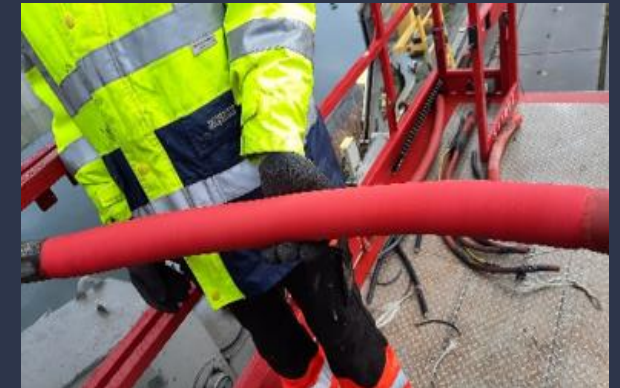
Repaired cable – fit for use
