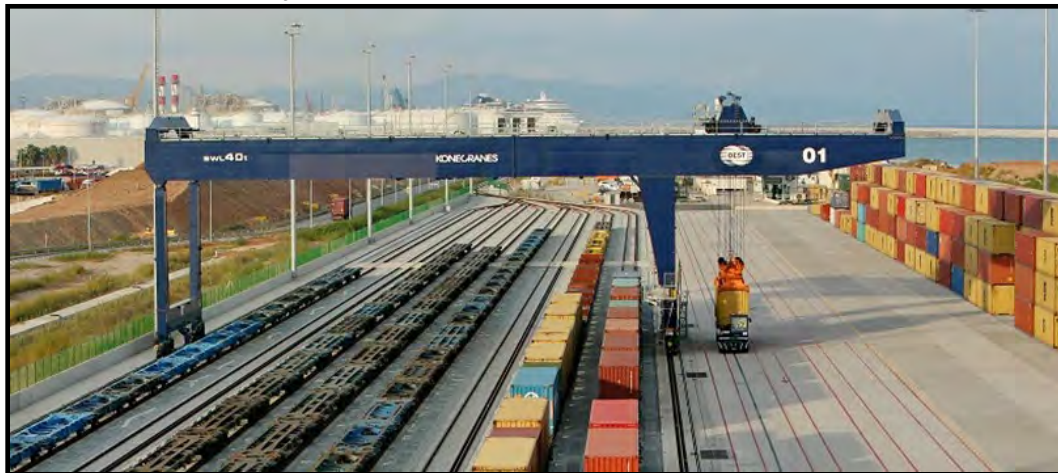
Wide Span Rail Mounted Gantry Cranes
