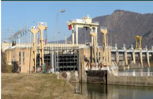
Upgrade of Iron Gate I Lock
