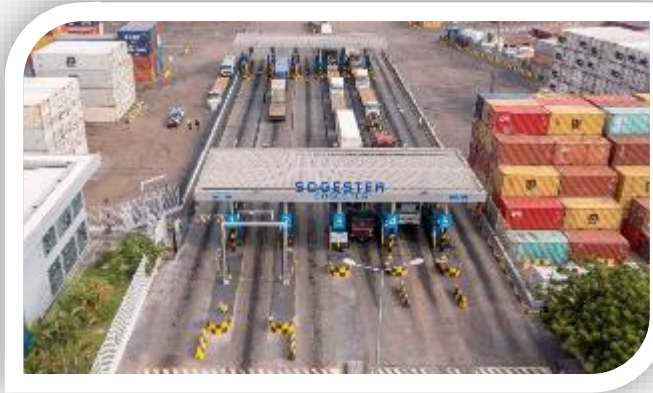
Gate Automation Camco OCR system (pilot Go-live)
