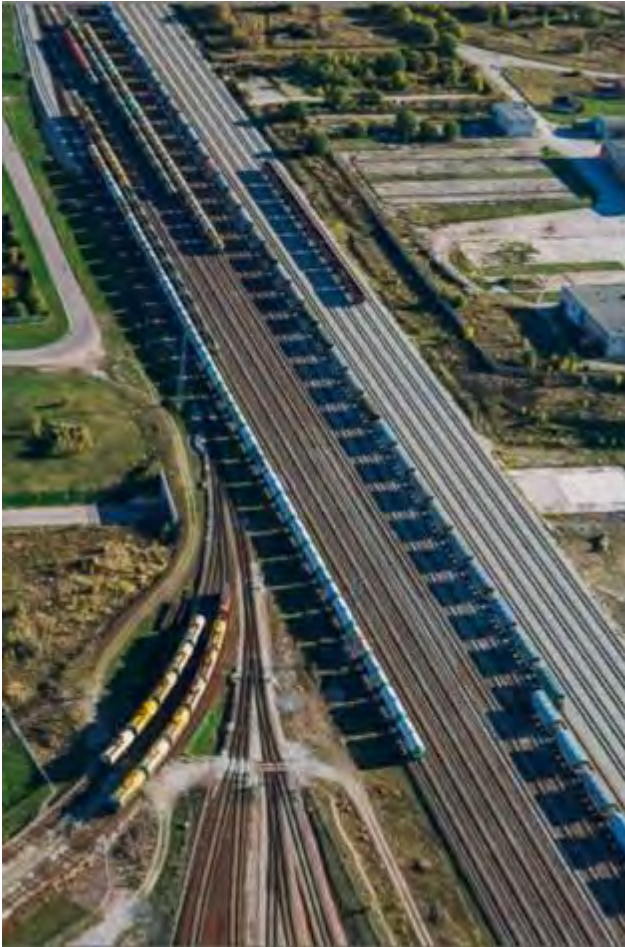
Silport upper railway station
