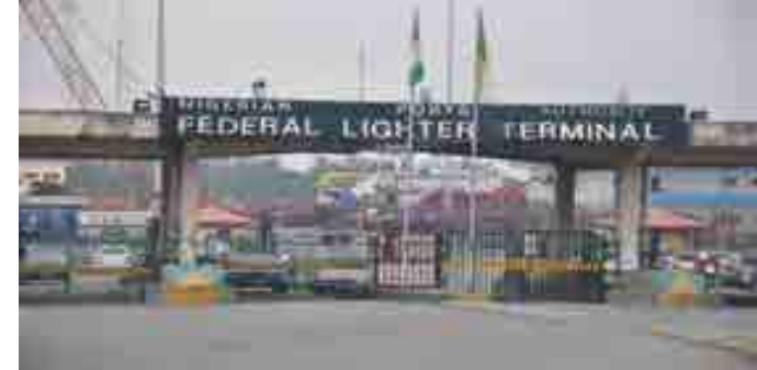
Onne Port Complex
