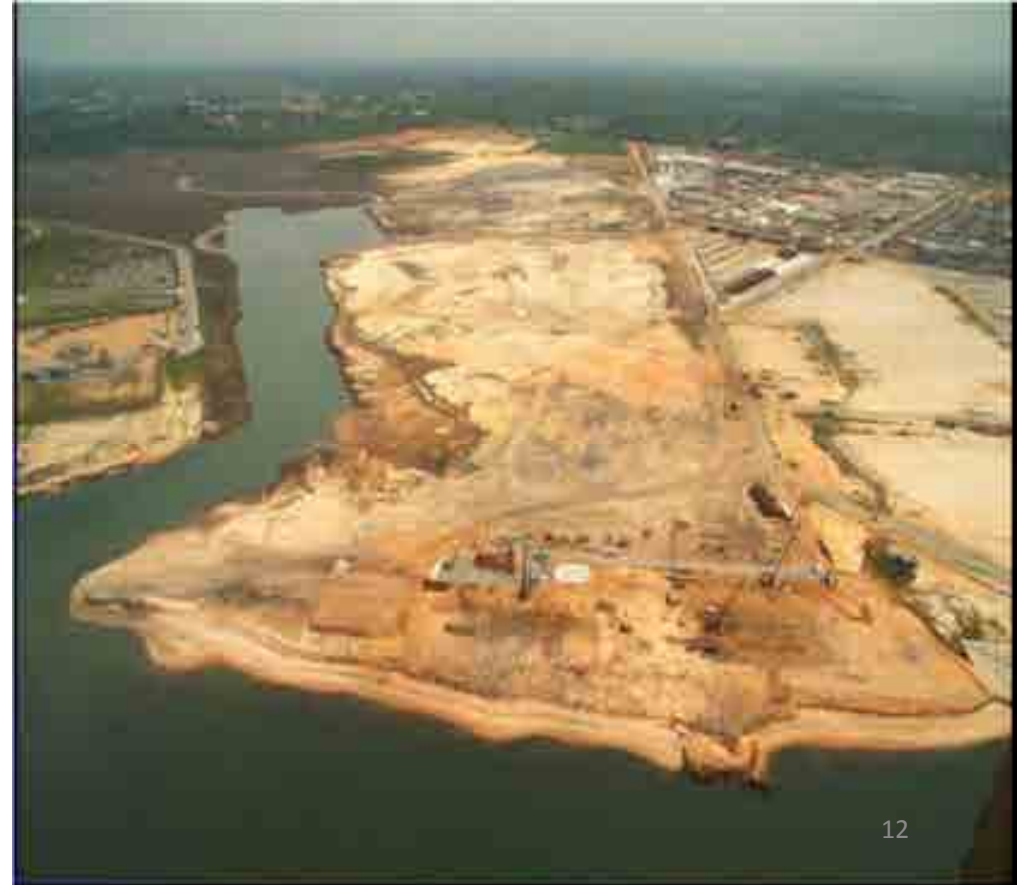
During Piling – Feb. 2006
