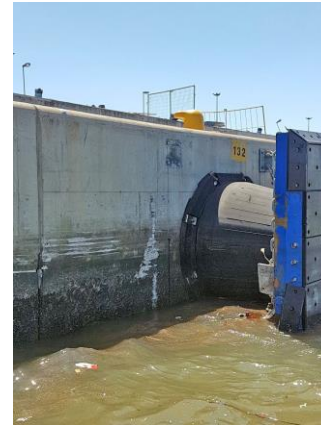
after floating crane collision
