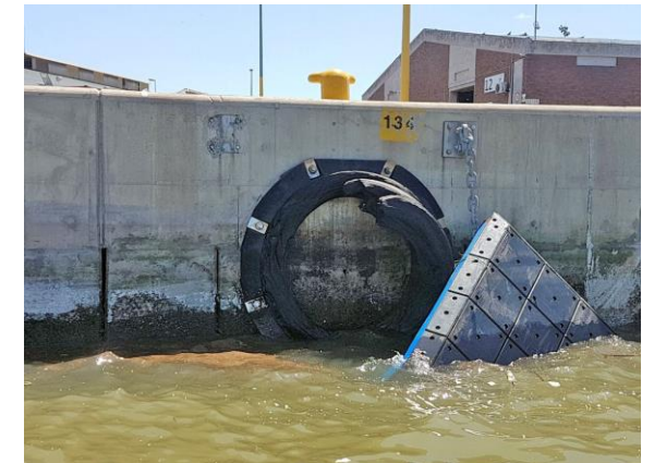
after floating crane collision
