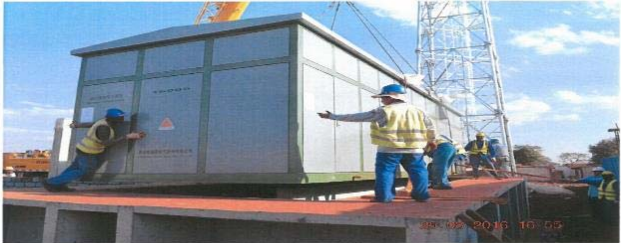
P9: Substation Installation of Section 9 (25 August, 2016 DK348)
