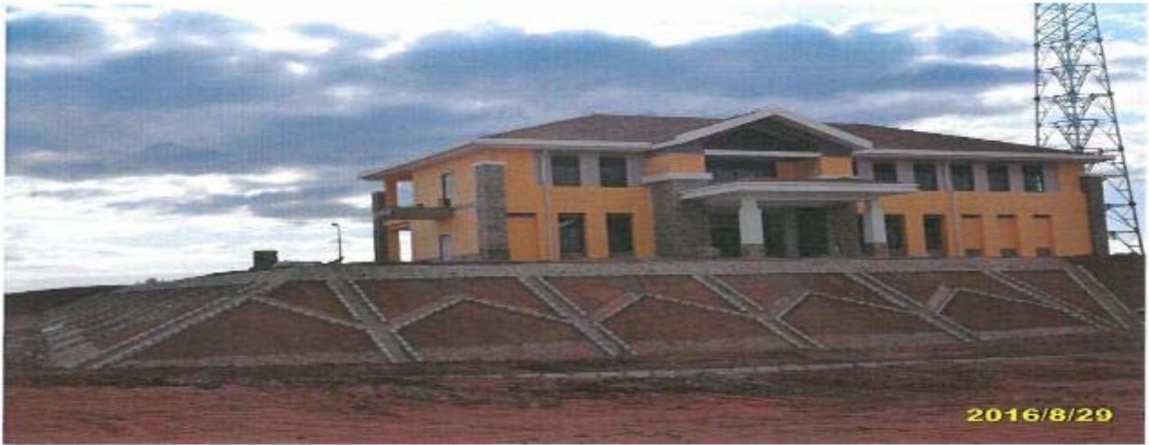
P3: Side slope protection of Section 3 (29 Aug 2016, DK251+500)
