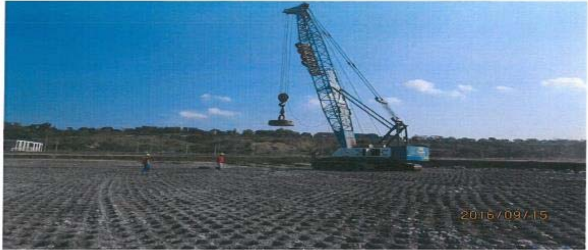
P1: Rvetment of Port Reitz Station of Section 1 (15 Sep 2016)
