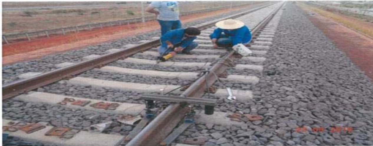
P7: Testing of track of Section 7 (23 Sep, 2016 DK352+000)
