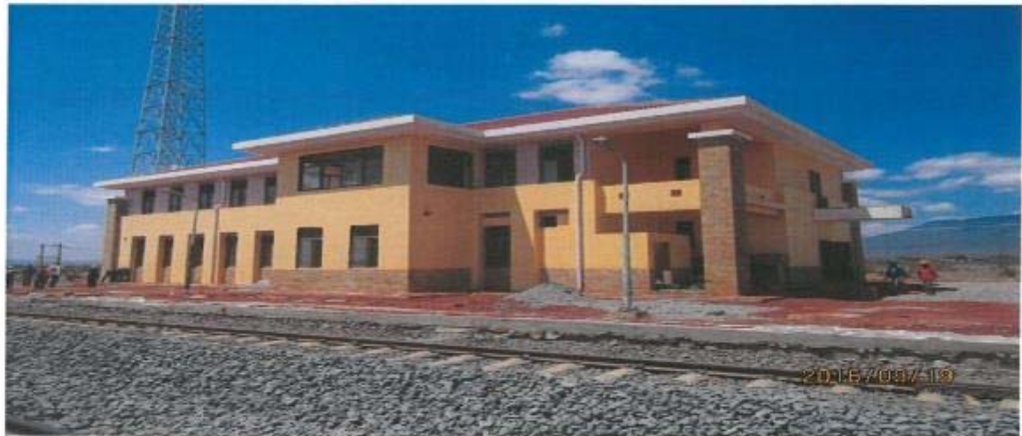
P2: Mackinnon Road Main Building of Section 2 (19 Sep. 2016, DK82+200)
