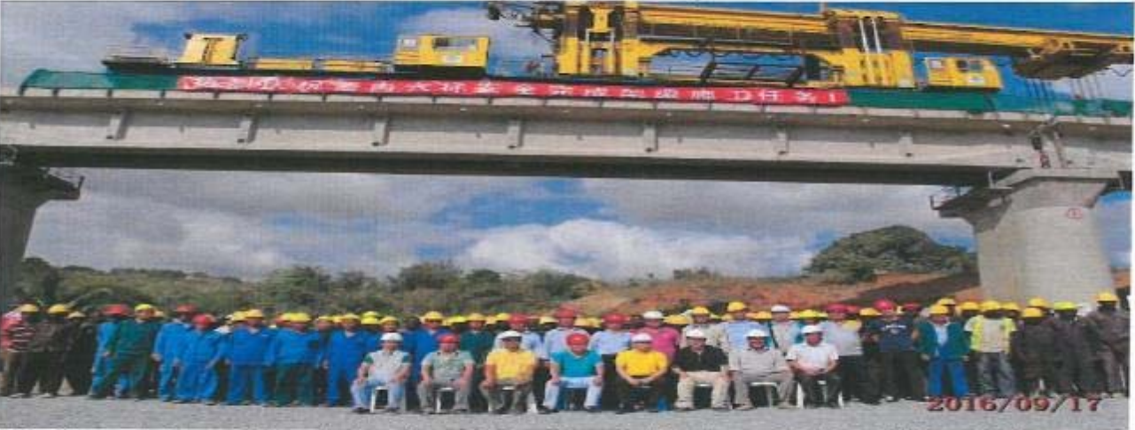
P6: Completion of Track Laying of Section 6 (17 Sep, 2016 DMK5+052)
