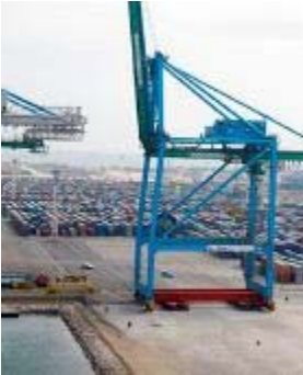
Marseille, France Upgrade of three non-Kalmar STS cranes ▪ Gantry upgrade ▪ SPMT relocation ▪ Electrical modifications
