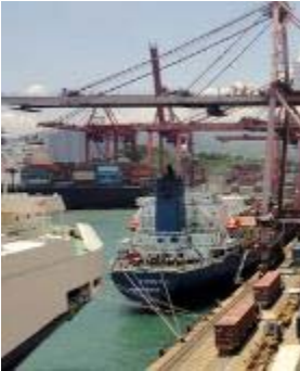
Hong Kong Structural visual inspection of four non-Kalmar STS cranes
