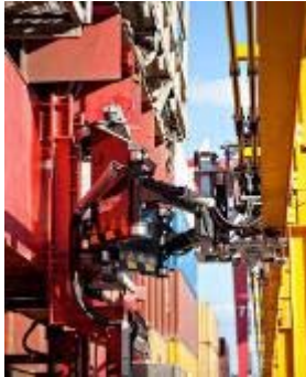
Yilport, Turkey Electrification of 18 non-Kalmar RTGs ▪ Installation and commissioning of pneumatic actuated automatic drive-in units ▪ Conductor bar system
