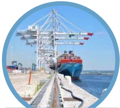
STS Crane Runways and Trolley
