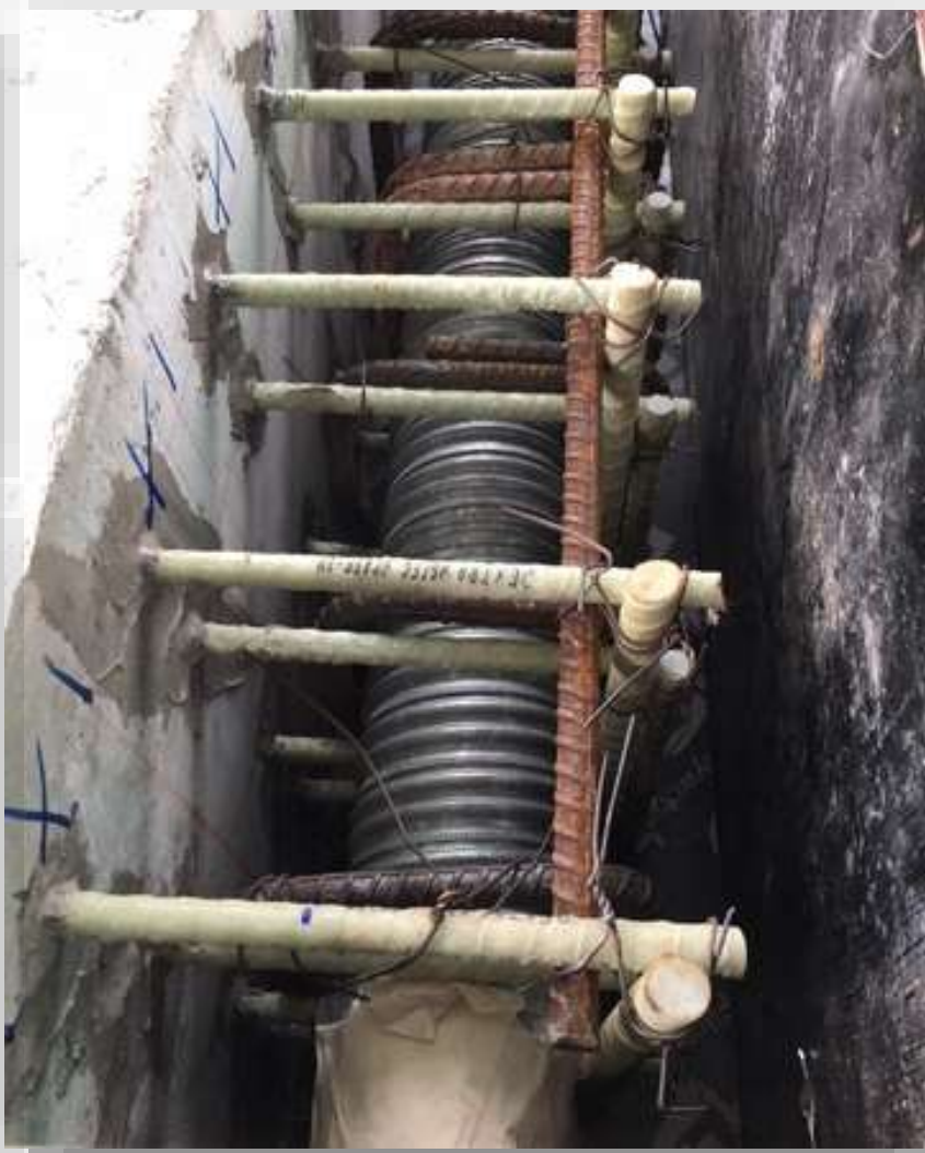
Concrete with GFRP dowels & post-tensioned steel bar
