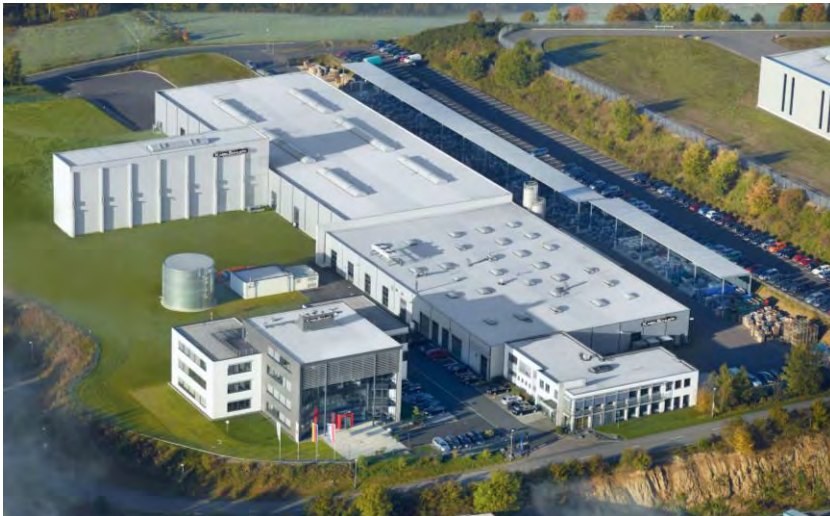
TSUBAKI KABELSCHLEPP Headquarters Wenden, Germany
