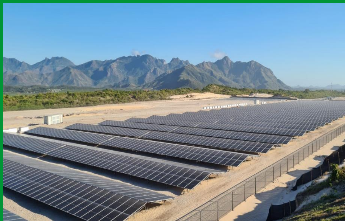
8 MW solar plant (Operational janv 2023)
