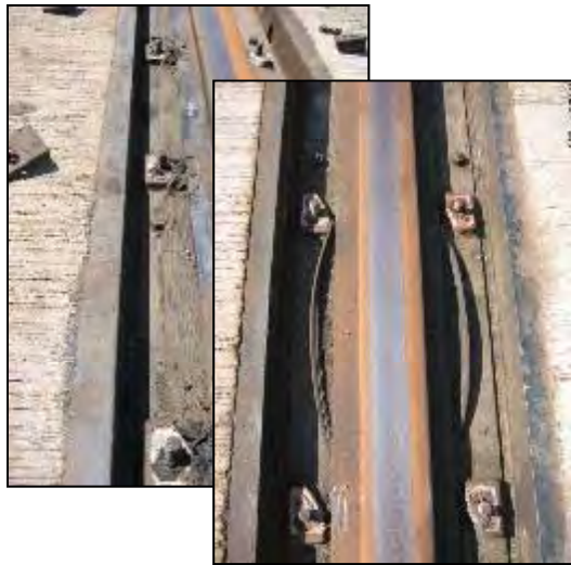
STS TRACK, HONG KONG
