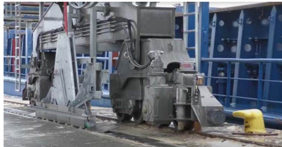
closed cable channel
