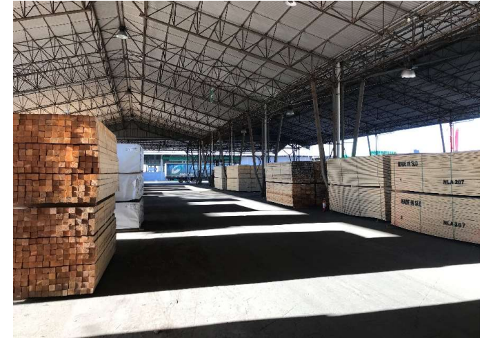
Sawn wood storage at former GCT terminal for regional exporters
