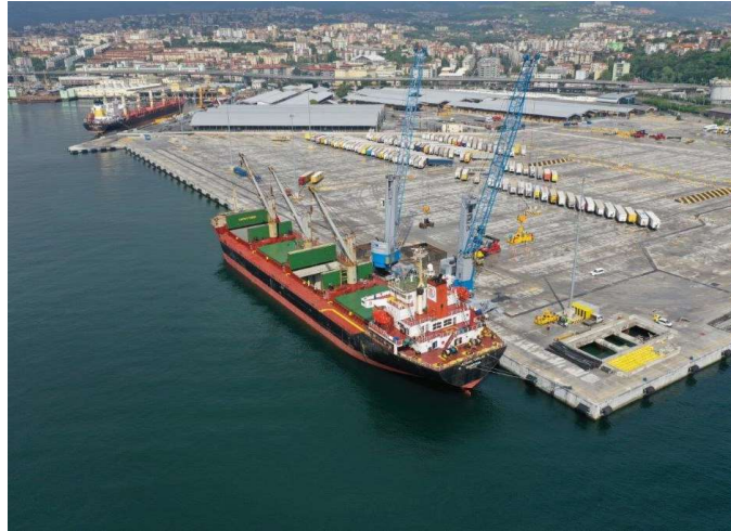
Pig iron unloading for neighboring steel mill
